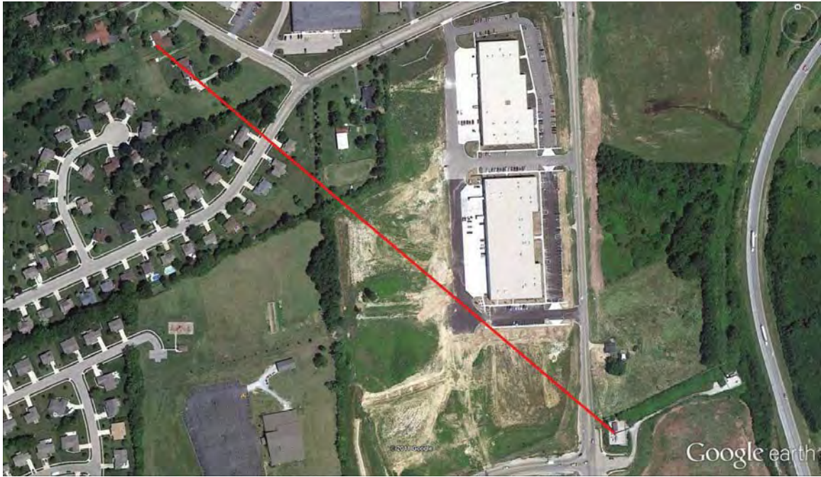
Figure 5. Satellite image of Transmitter to Receiver path. The path length is 623 m. The distance from the KILN radar (not shown) is 42 km. Image copyright owned by ©Google 2011.
